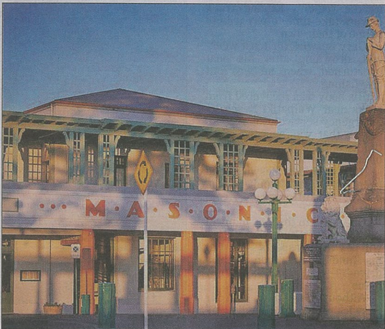
FINE BUILDING: The Art Deco Masonic Hotel was described as the key to a full Art Deco experience.
